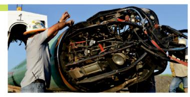
External GMAW/PGMAW root welding utilizing Copper Back-up Clamps (CBUC)
